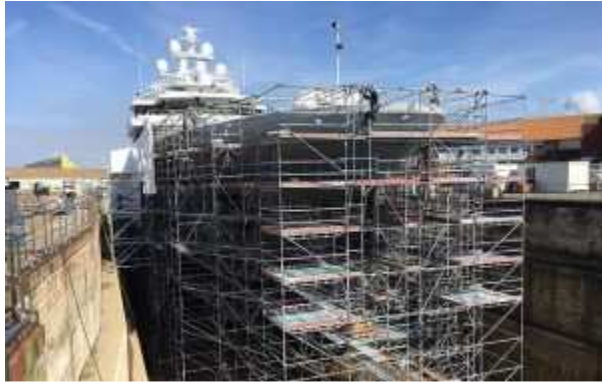
Compositeworks refit project in La Rochelle
